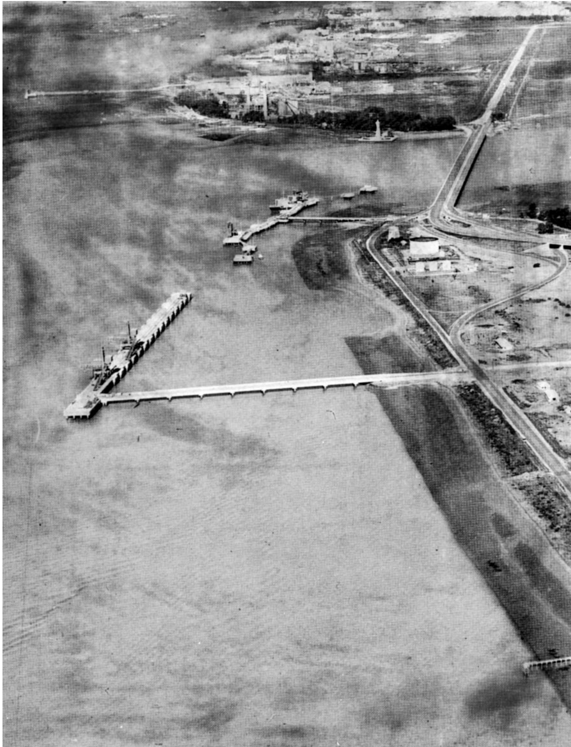
Huelva—Petroleum and Mineral Piers
