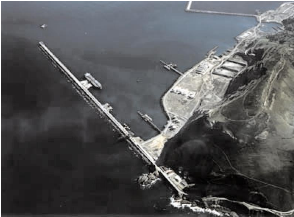
Bilbao—Punta Lucero Breakwater from W
