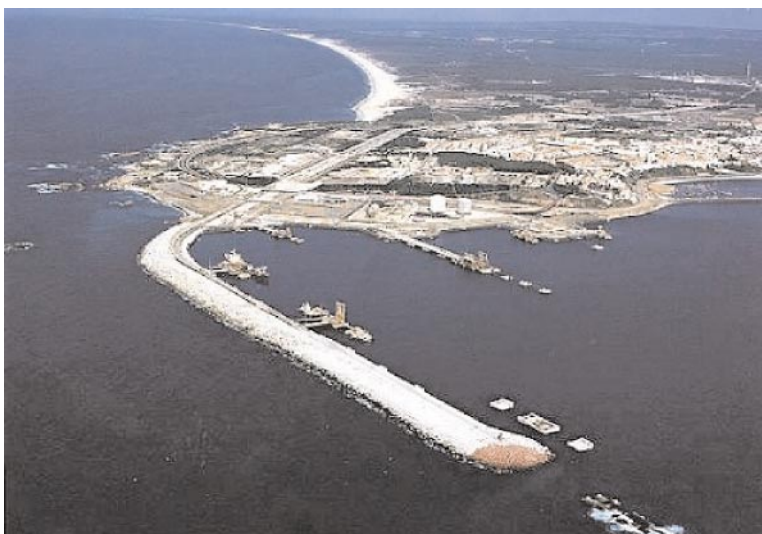
Sines—Oil and Petrochemical Terminal
