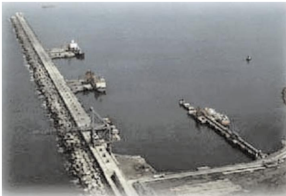
Bilbao—Punta Lucero Breakwater from SSW
