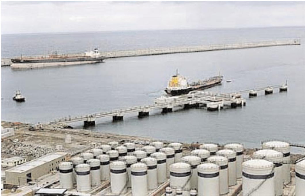
Bilbao—Punta Lucera Breakwater from SE
